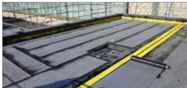
Simple sandwich installation between two geomembranes
