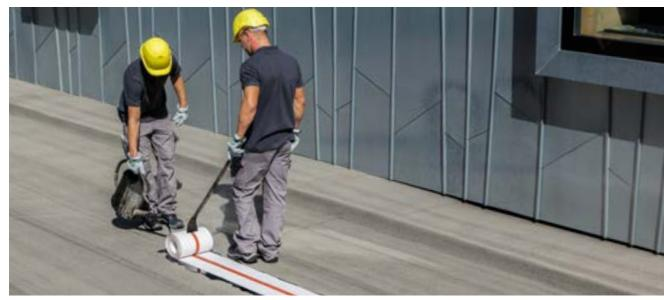
RedLINE® expansion joint strips are generally delivered prefabricated with all preforms on a project-specific basis. For installations in several stages or for very long building joints that make handling more difficult, the specially developed vulcanization device can be used to produce the strip on site. Ask our technical services department directly about the options available (info@soba-inter.com).
