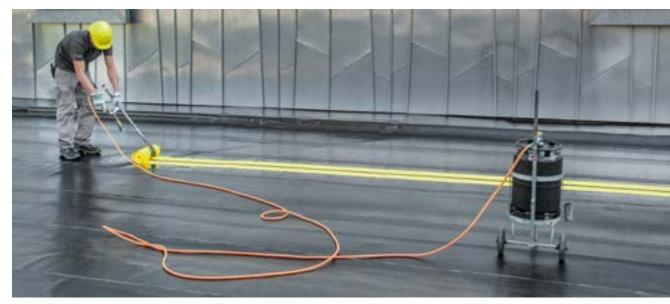
FlamLINE® expansion joint strips are generally delivered prefabricated with all preforms on a project-specific basis. For installations in several stages or for very long building joints that make handling more difficult, the specially developed vulcanization device can be used to produce the strip on site. Ask our technical services department directly about the options available (info@soba-inter.com).
